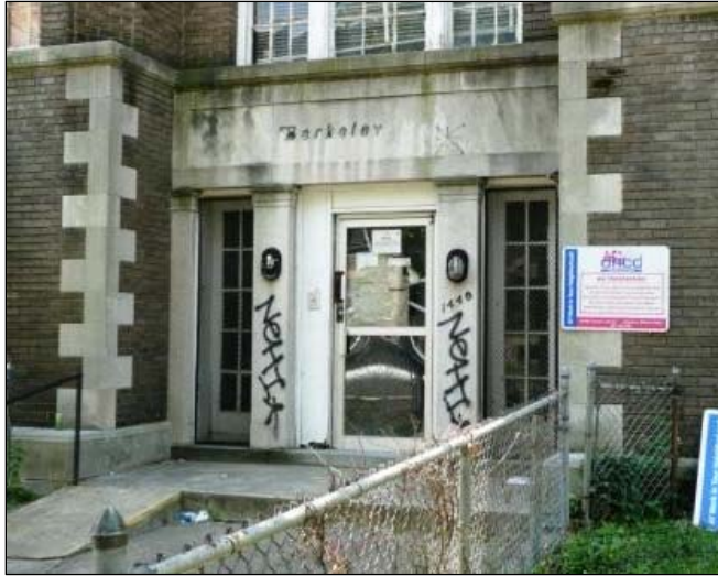
Before CityPartners Renovation
